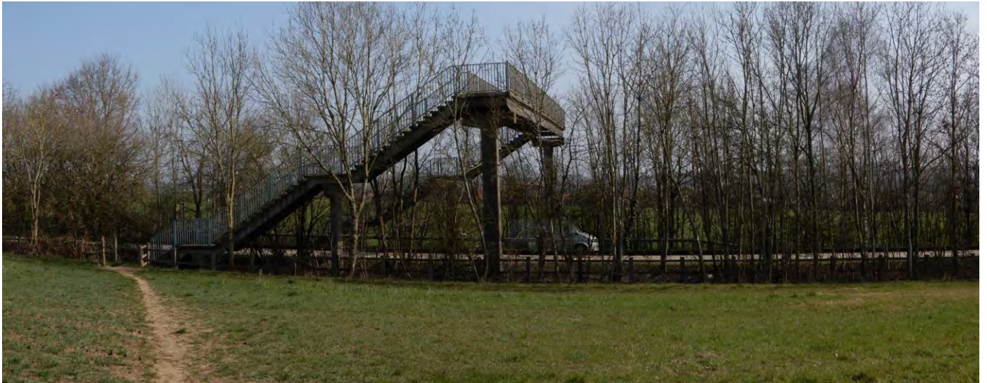
41. View along the line of Footpath Aspenden 001 from the west side of the A10 - the footbridge (and also to a lesser extent the site beyond it) can be seen through the trees in the winter. Three images combined, March 2022.
