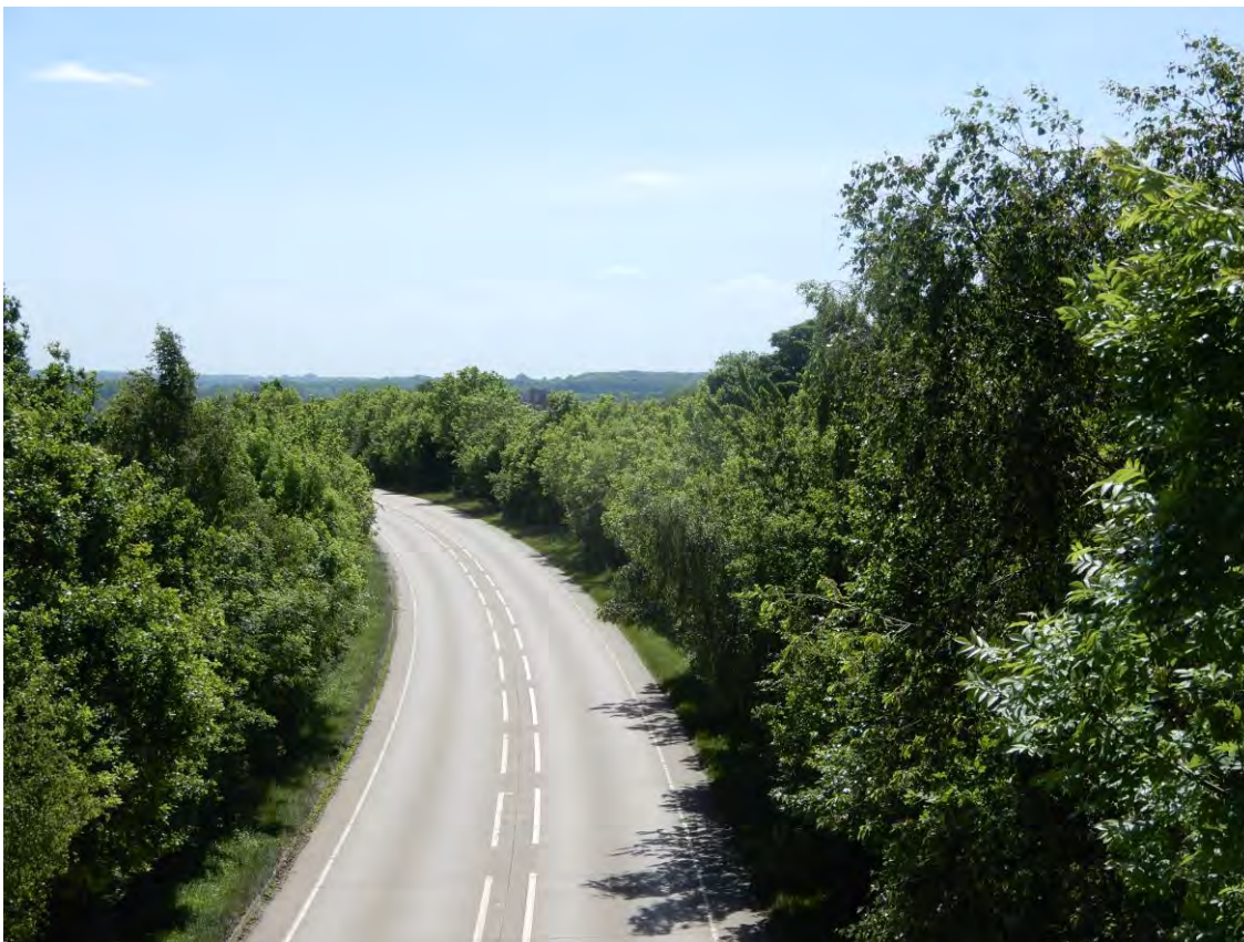
43. View south along the line of the A10 from the footbridge - the road forms an effective screen and break in the local landscape, especially in the summer. May 2022.
